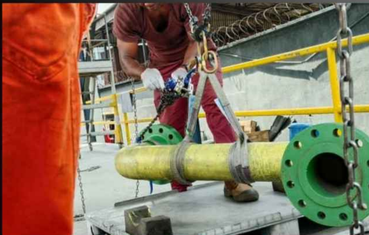
Pipe Fabrication and maintenance I
